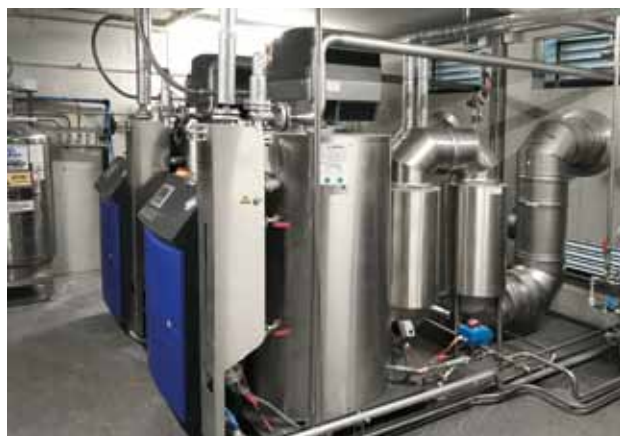
Fig.: Multiple unit. Second downstream JUMAG economiser installed space-savingsly on the basic frame
