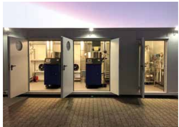
Fig.: Container steam system
